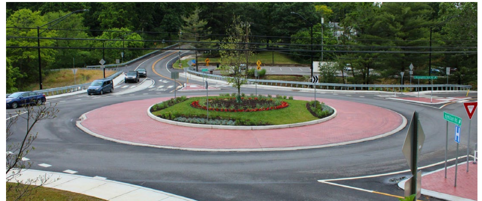
The award-winning 2022 McLaughlin Run Road roundabout, image courtesy of Upper St. Clair
